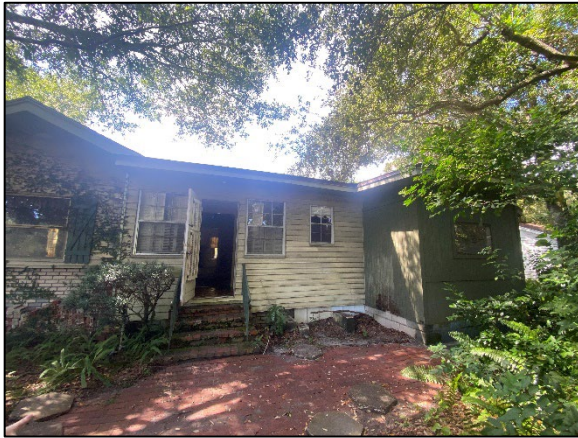
Figure 4: East elevation of primary residence, showing enclosed porch (center) and c. 1975 addition (right), which are proposed for demolition
